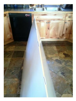
6. Place 3 soft 1 ½" pieces of hooked Velcro on both angled ends of each base board. Note: when cutting board, make sure there is enough wood to allow for loss of length, and make sure the beveled edges are facing opposite ways on opposite ends of each board.
