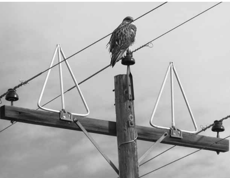
Figure 4. Perch deterrents minimize electrocution risks, but potential perch sites remain.
