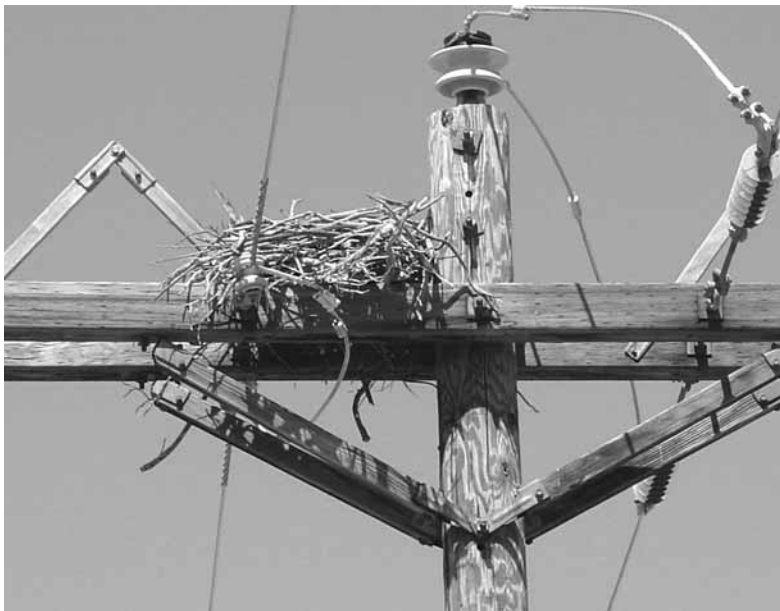
Figure 7. Raptor nest on a structure fitted with anti-perching devices (Tri-State G&T).
