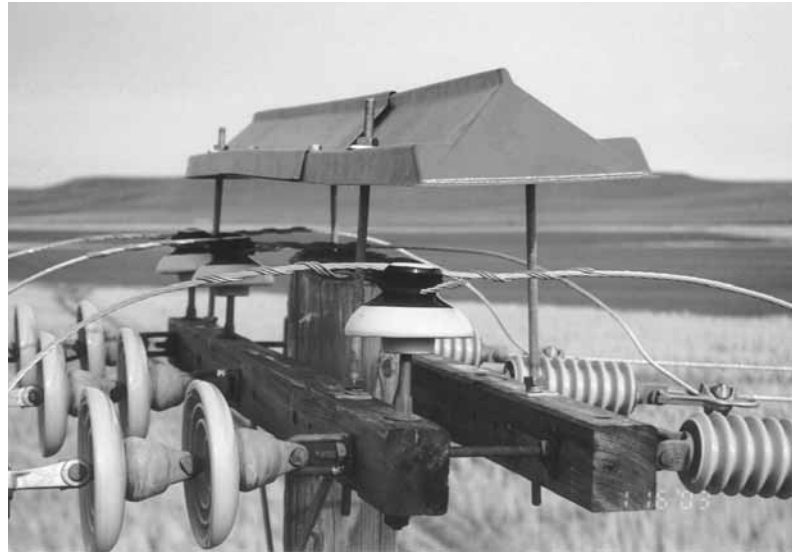
Figure 6. Stick deflector at a double dead-end structure (Kaddas).
